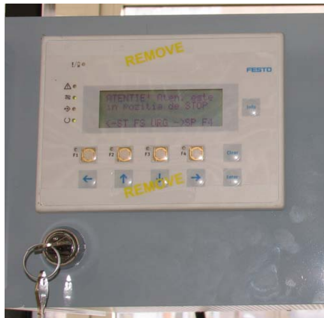
Figure 3.6 PLC Cubicle- Operator Unit (OU)
