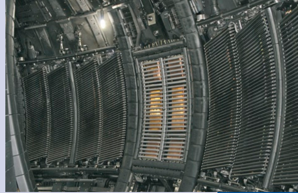
The ITER-like Antenna ILA (installed in 2007, 7.2MW, 0.9m 2 ) between two A2 antennas (1996, up to 4MW, 2.2m 2 ) inside JET. The copper coloured areas behind the bars of the Faraday Screen are the straps of the ILA. (Photo: EFDA JET)
